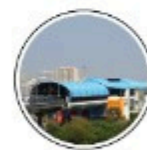
Adjacent to City Center Metro Station
