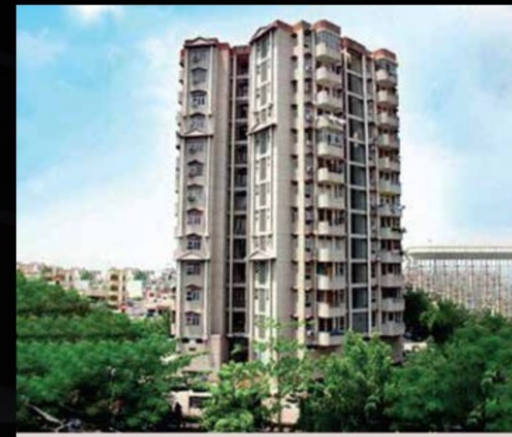
Devika Apartments, Ghaziabad
