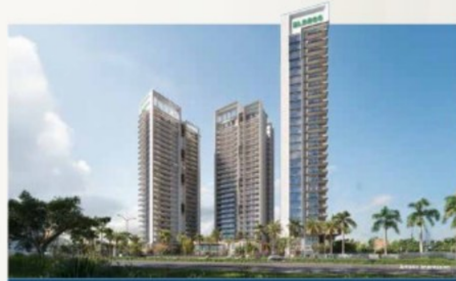
Eldeco Trinity, Gomti Nagar Extension, Lucknow
